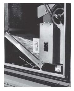
"N3" - Flush Mounted Disconnect Switch and GFI Convenience Outlet
